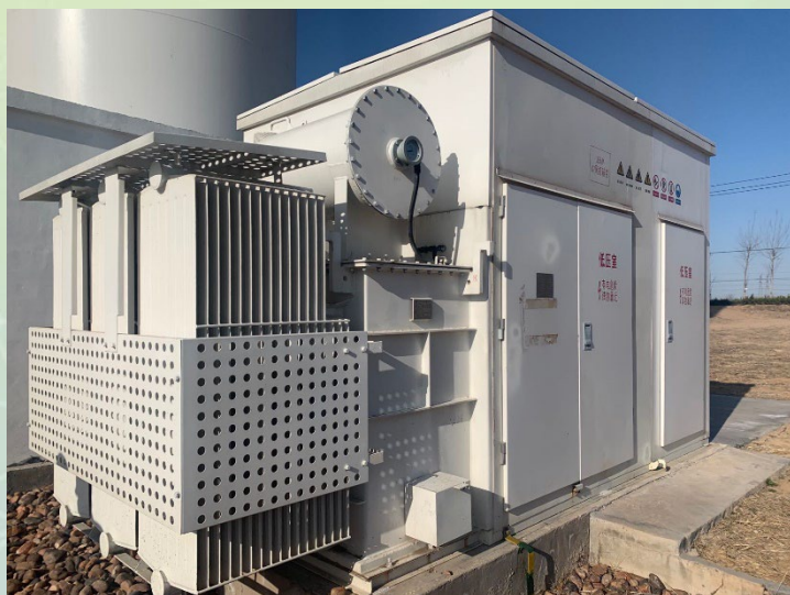
5500 kVA wind power step-up amorphous transformer
