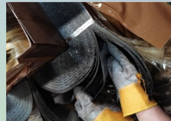
Amorphous transformer core replacement
