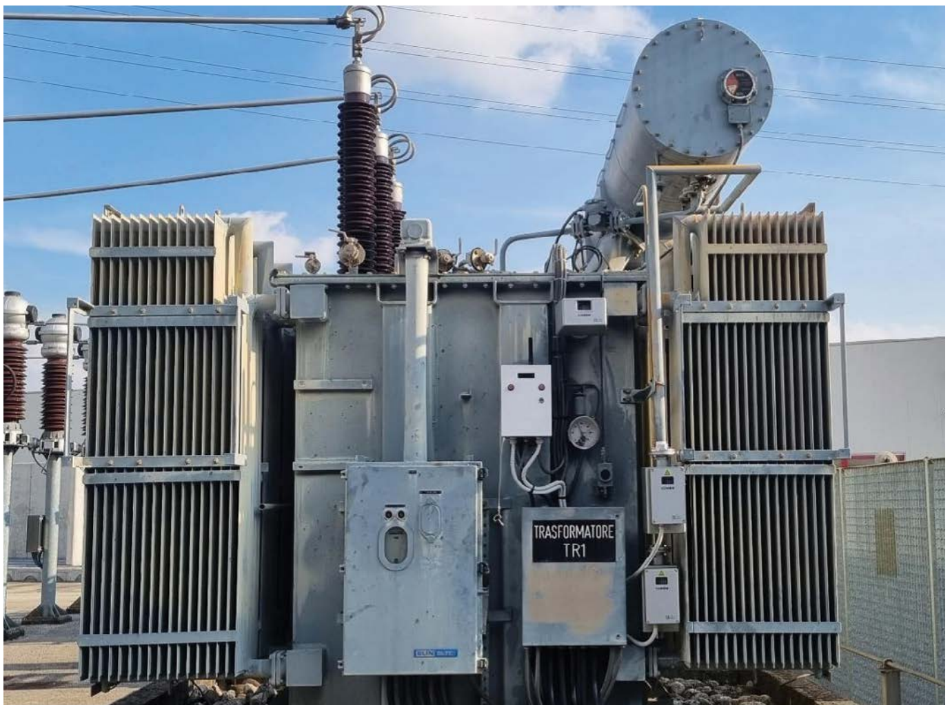
Smart accessories enable continuous and remote monitoring and data gathering of transformer health.
