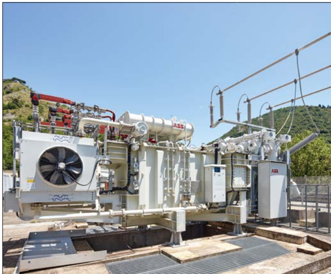
Figure 6. Power transformers for mobile substations can be easily arranged in many configurations, mounted for air, rail and road transportation and installed almost anywhere.
