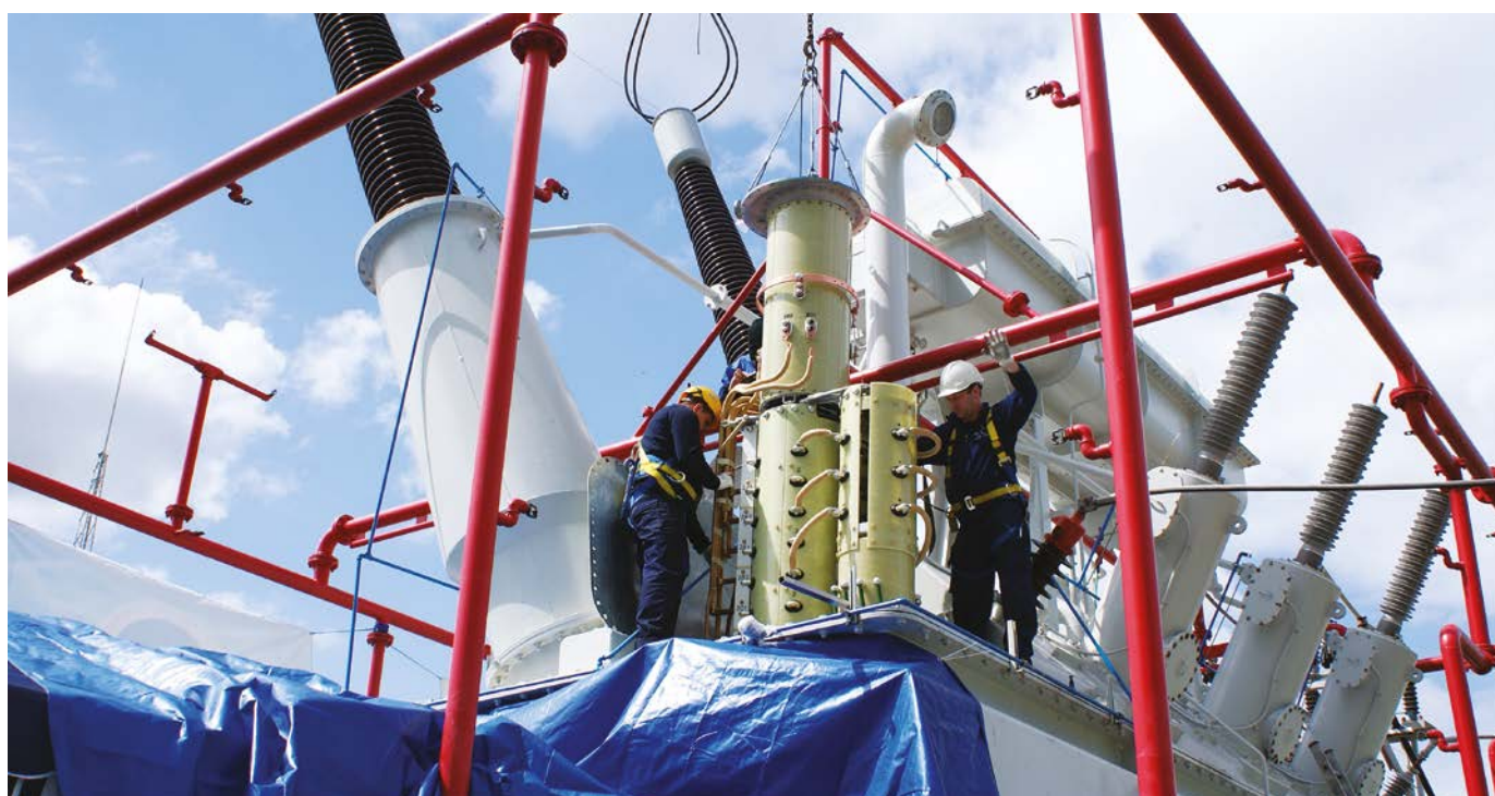
Figure 4. OLTC replacement in a transformer on site
