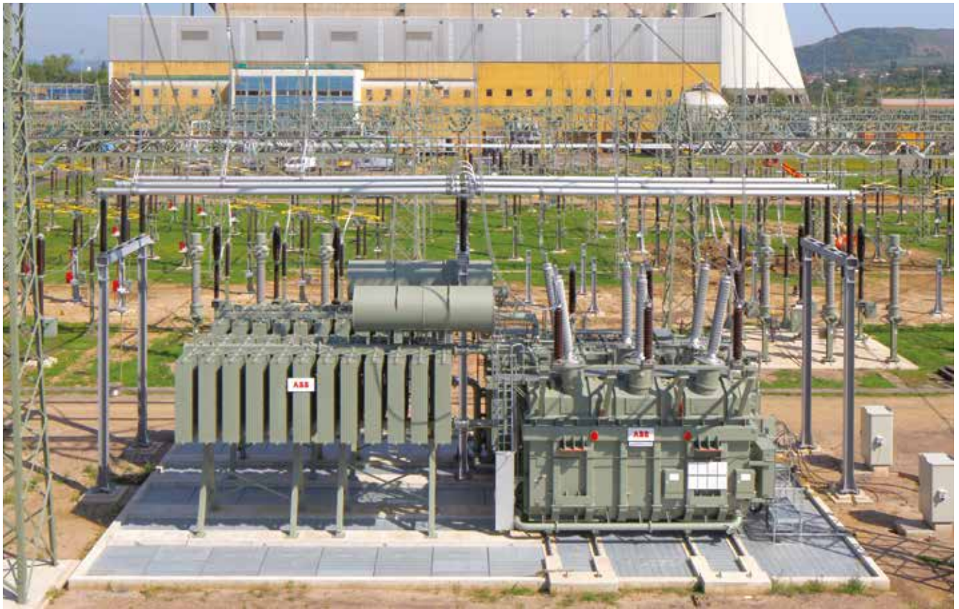
Figure 4. Phase-shifting transformer
