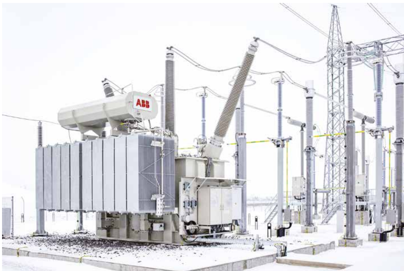
Figure 1. Shunt reactor
